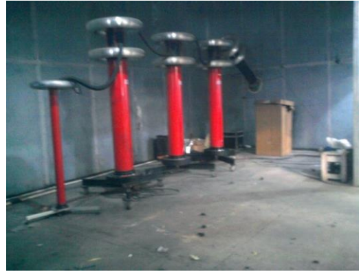
Fig 6: Partial Discharge Lab HV Transformer and Coupling and blocking capacitor with Inductor with toroide.
